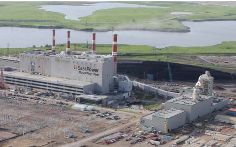
SaskPower Boundary Dam carbon capture and storage.
